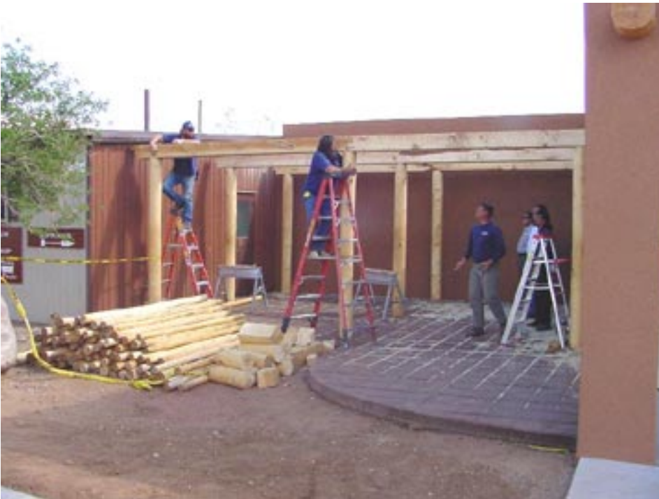
New Patio under construction at Museum
