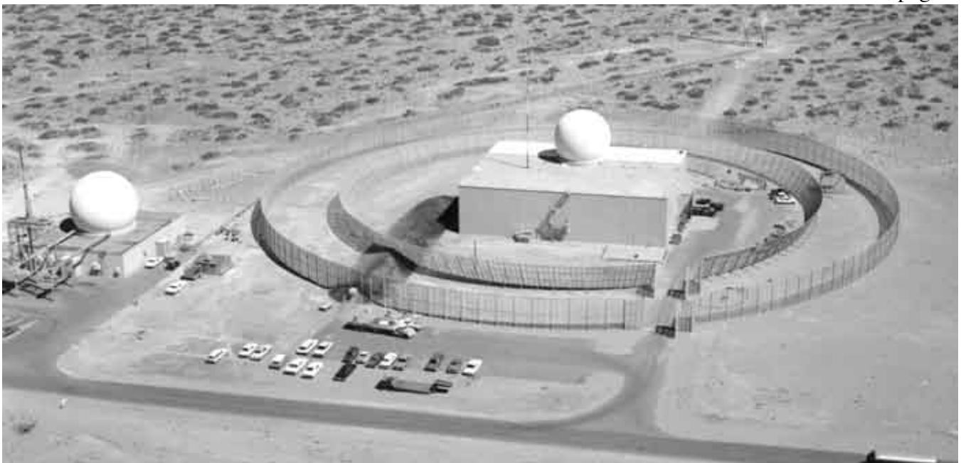
This photo shows the Target Tracking Radar (TTR) on the left and the Discrimination Radar (DR) at right.
