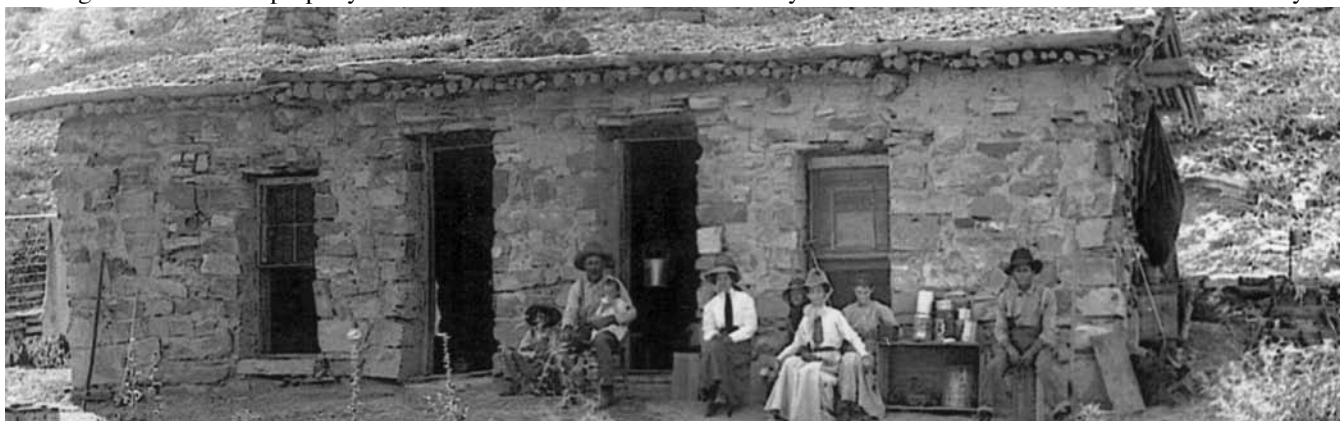
The Garrett Bear Canyon house that was supposedly needed to smuggle Chinese north. The house walls are still standing but many years ago WSMR paid Human Systems Research to stabilize and put a new roof on it. The photo was taken sometime after Pat Garrett owned the place.
