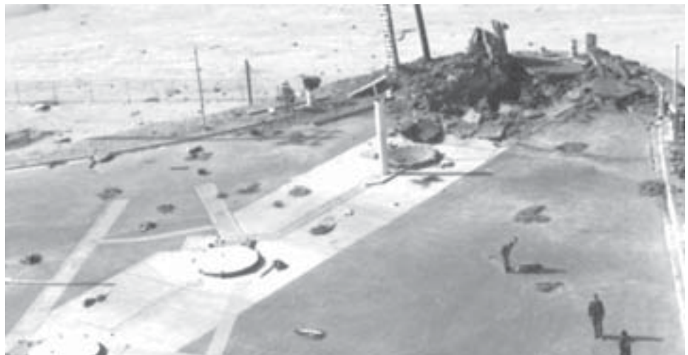
Damage to Sprint launch cell at LC-50 from missile explosion on March 15, 1966.
