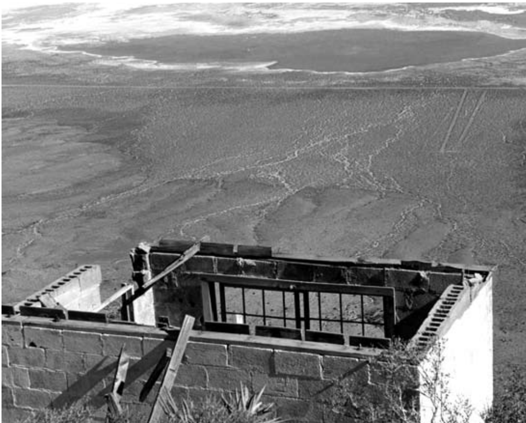
Taken in 1986 this photo shows the shelter building at the top of the peak with its roof blown off. At the top of the photo is Lake Lucero to the east. The straight line crossing the photo just below Lake Lucero is Range Road 7. (Eckles photo)
