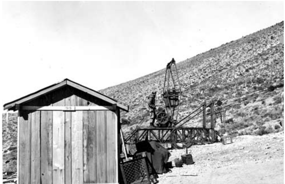
Above is a closeup of the gauges and key for the engine that pulled the moveable cable on the tram. At right, this 1948 photo shows a soldier manning the engine mounted in the bottom framework. The building, numbered 1919, housed maintenance parts and equipment for the system. All of these things were still there in 1986.
