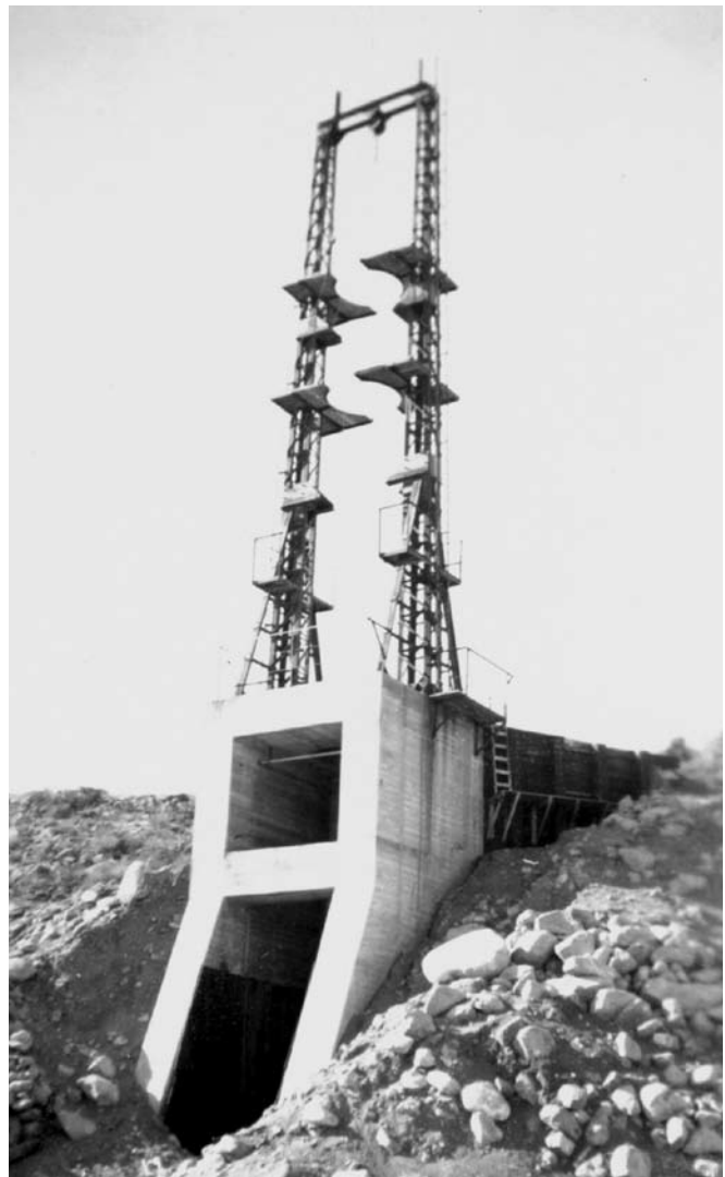
Newly constructed 100K Static Test Stand in 1946.
