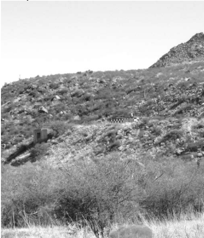
Remains of the 100,000 Pound Static Test Stand today with the black and white checkerboard block house.
