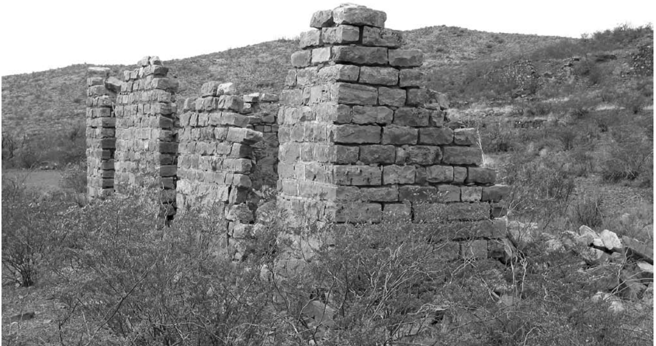
The walls to the assay office at Estey City still stand. Estey City was a small copper mining community in 1904 and dead by 1910. It is just east of the Oscura Mtns. and is the only real ghost town on WSMR. Photo by Jim Eckles
