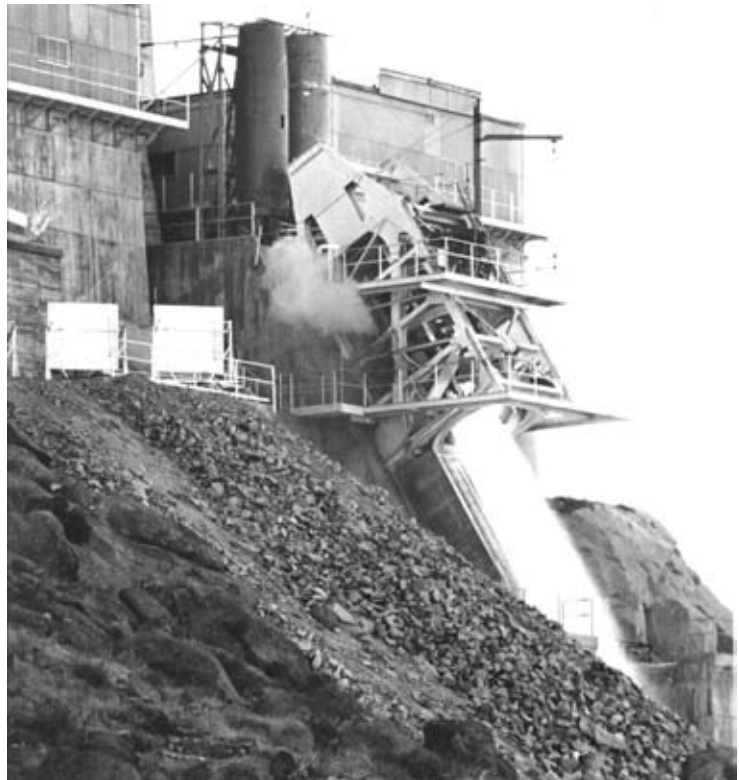
A Redstone engine test at 500K on Nov. 8, 1951
