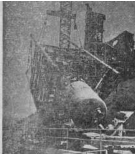
INTO POSITION AT WSMR — Tank and cage assembly for Redstone missile motor testing is unloaded from its trailer carrier and shifted into position at the 500,000 pound static test facility here. Hauling the huge assembly up the side of the Organ mountains to the test stand proved to be an engineering feat in itself.
